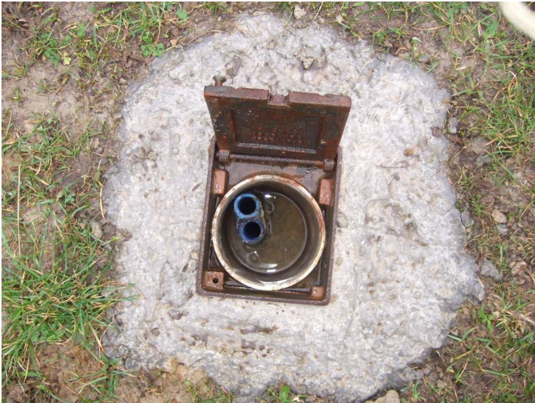
Plate 8 BH9 located at The Holms, Scarborough North Bay
