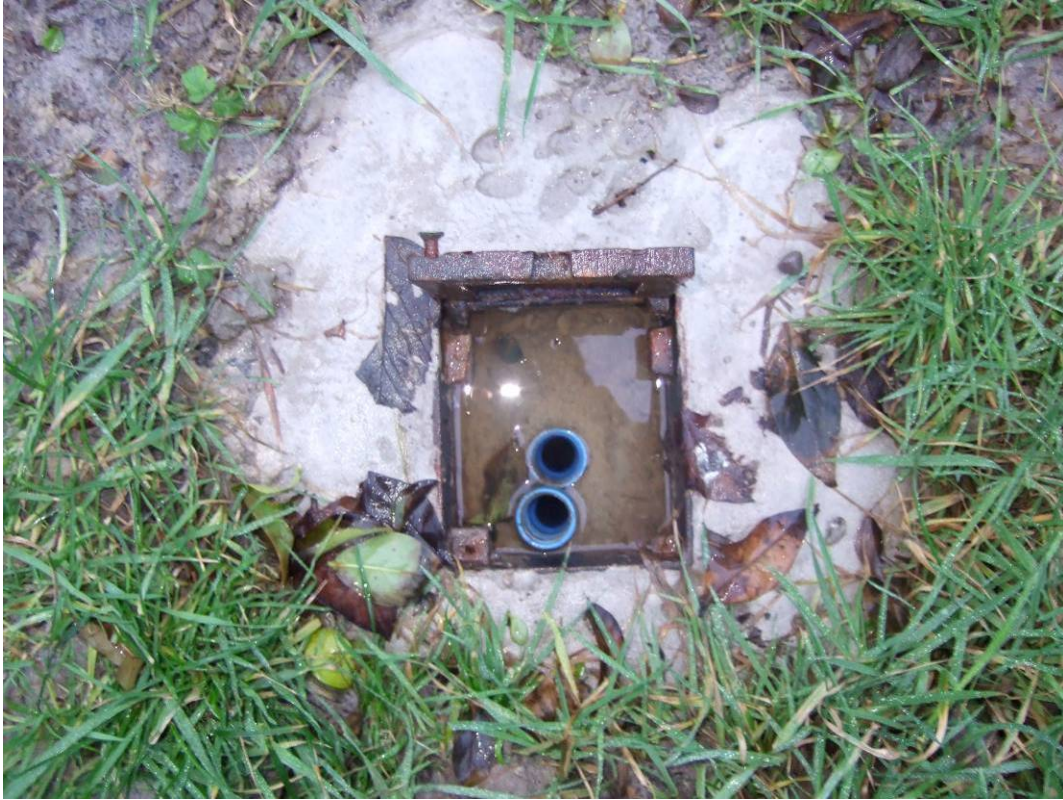
Plate 7 BH8 located at The Holms, Scarborough North Bay
