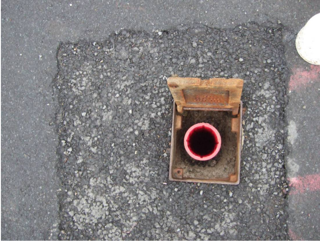
Plate 13 BH14 located on The Promenade above Spa Cliff
