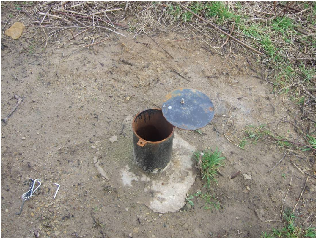
Plate 6 BH7 located at Scalby Ness
