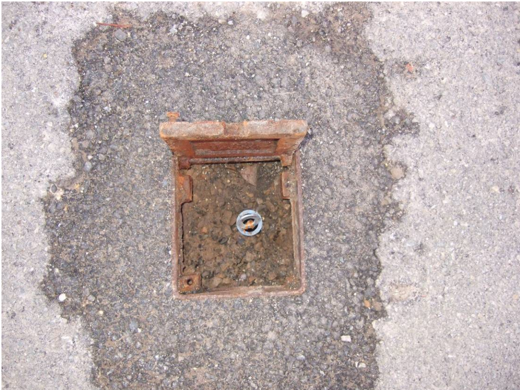
Plate 14 BH15 located landward of The Promenade above South Cliff Gardens
