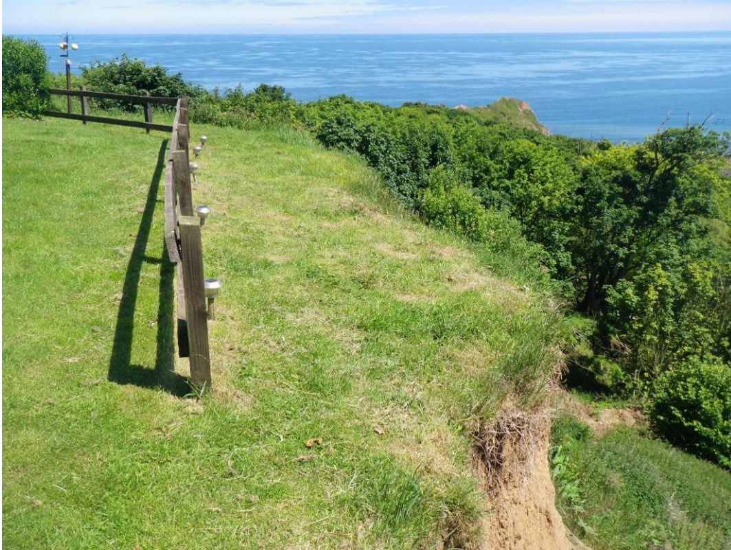
Plate 9 Cliff recession at Knipe Point Headscarp looking east (17 th June 2010)
