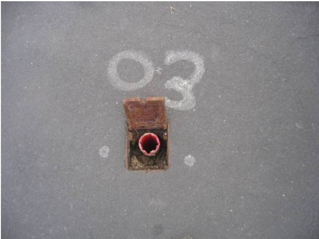
Plate 38 Scarborough South Cliff H6 (AA03)
