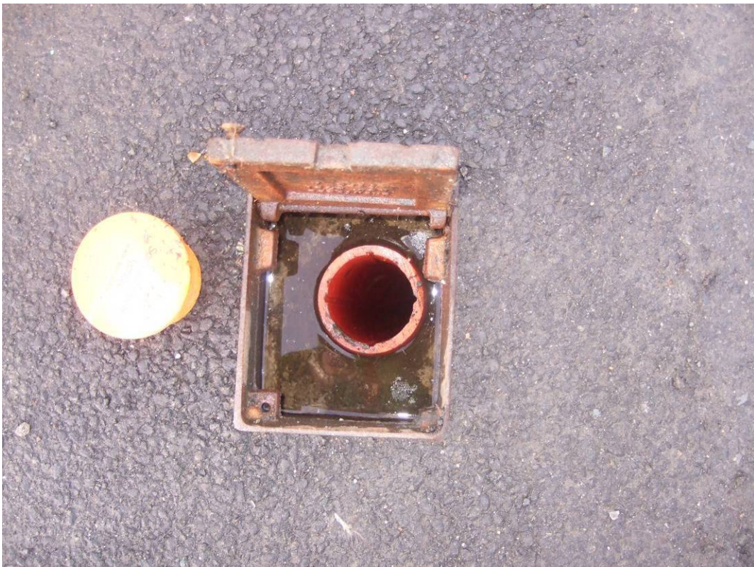
Plate 12 BH13 located on The Promenade above Spa Cliff
