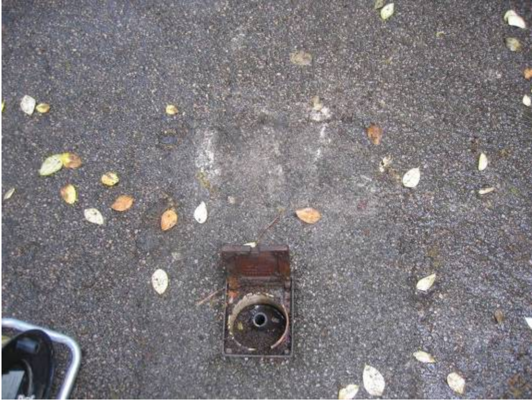
Plate 51 Scarborough South Cliff H5
