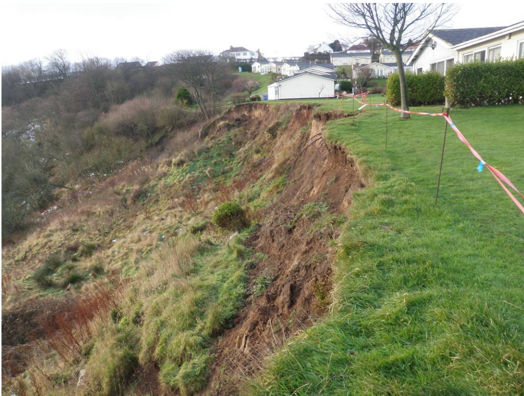
Plate 6 Cliff recession at Knipe Point Headscarp (13 th December 2010)
