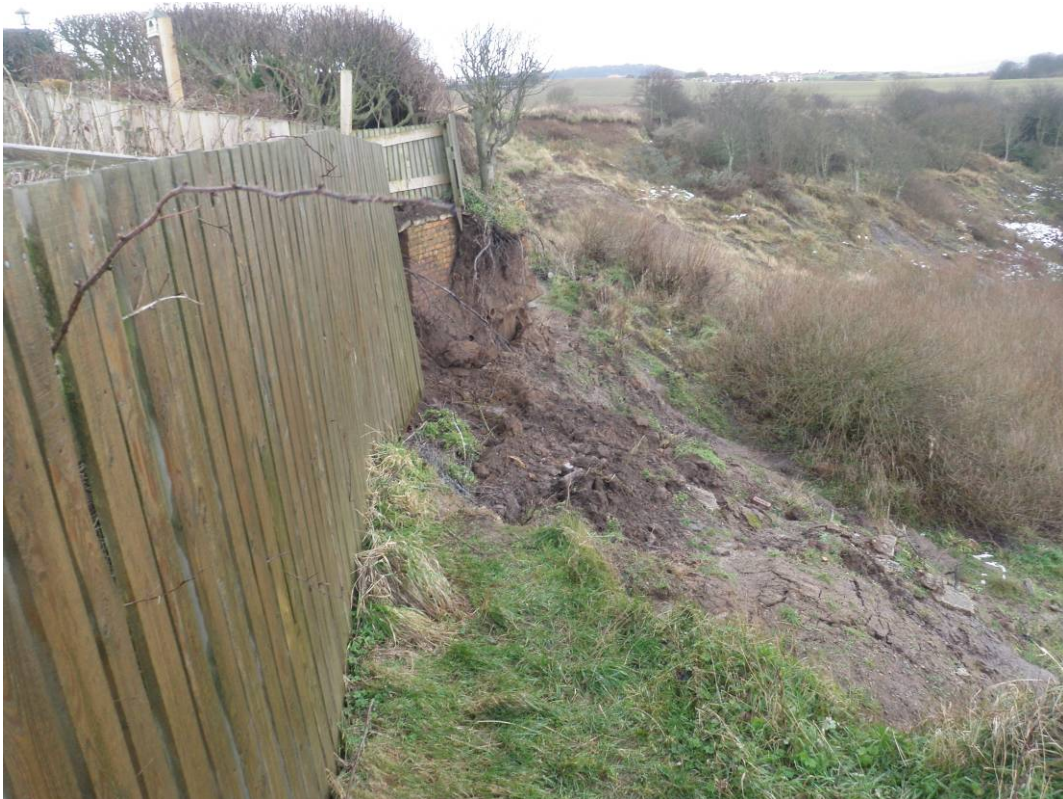
Plate 2 Cornelian Bay side of Knipe Point looking northwest (13 th December 2010)
