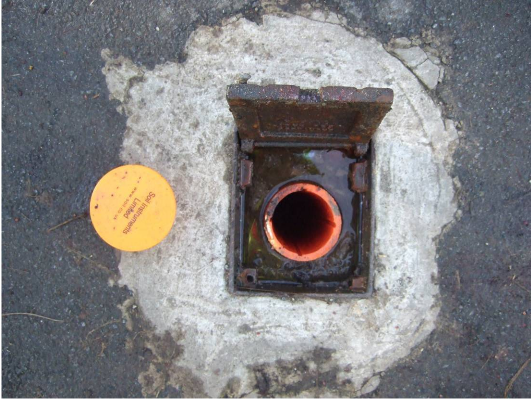
Plate 19 BH20 located mid-slope below The Rose Gardens
