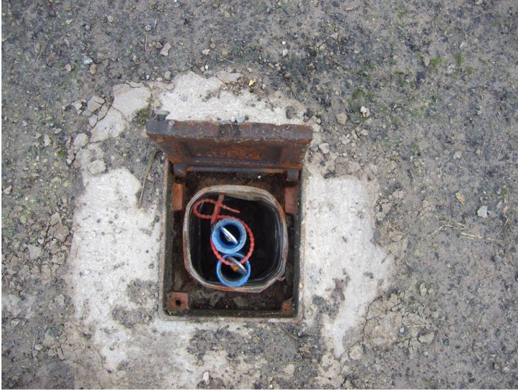
Plate 17 BH18 located mid-slope below The Rose Gardens
